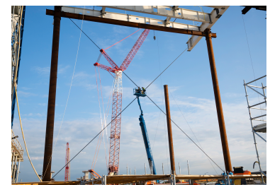
Temporary falsework for the back span
