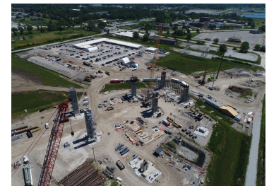
Side span piers and anchor piers
