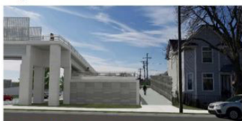
South View from Junction
