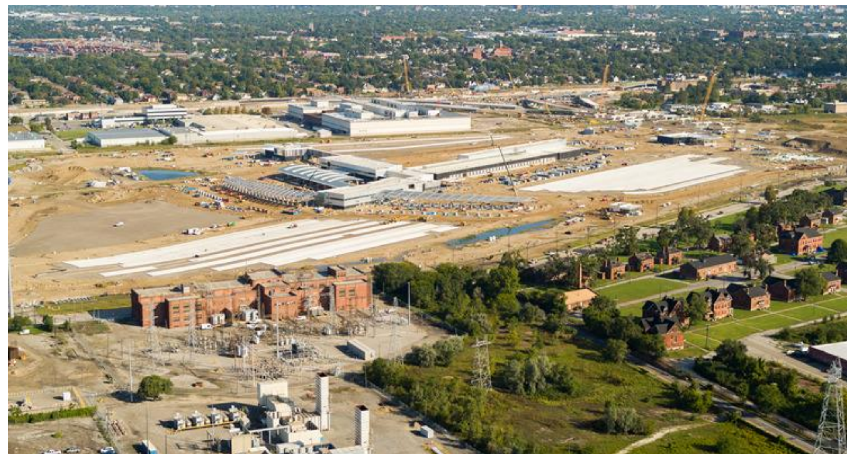
US Port of Entry construction progress
