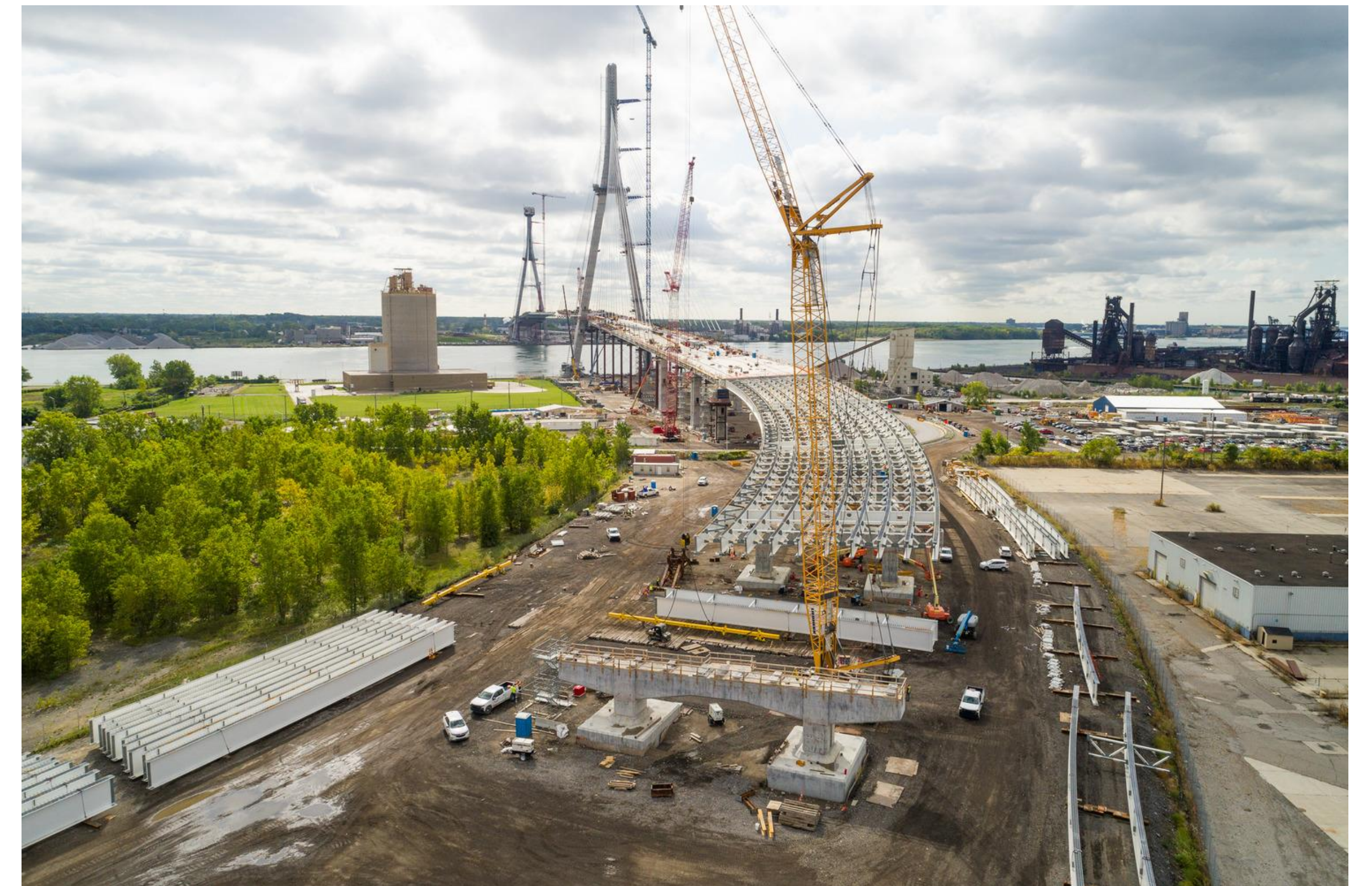
US bridge site construction progress.
