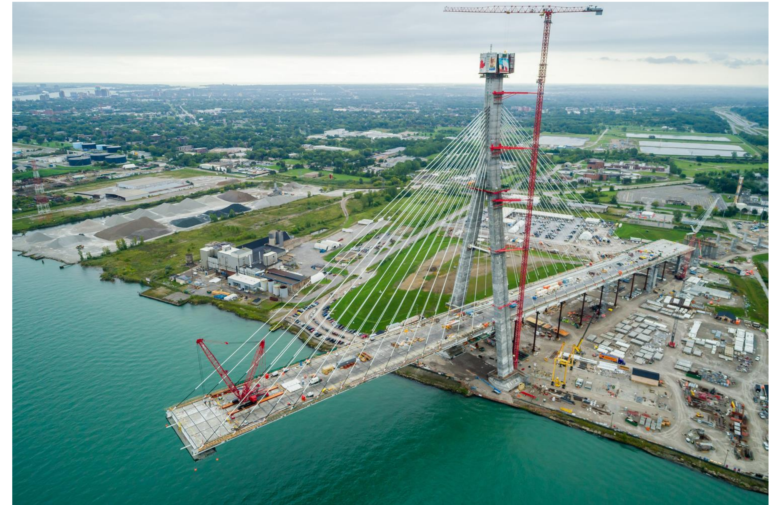
Canadian bridge site construction progress.
