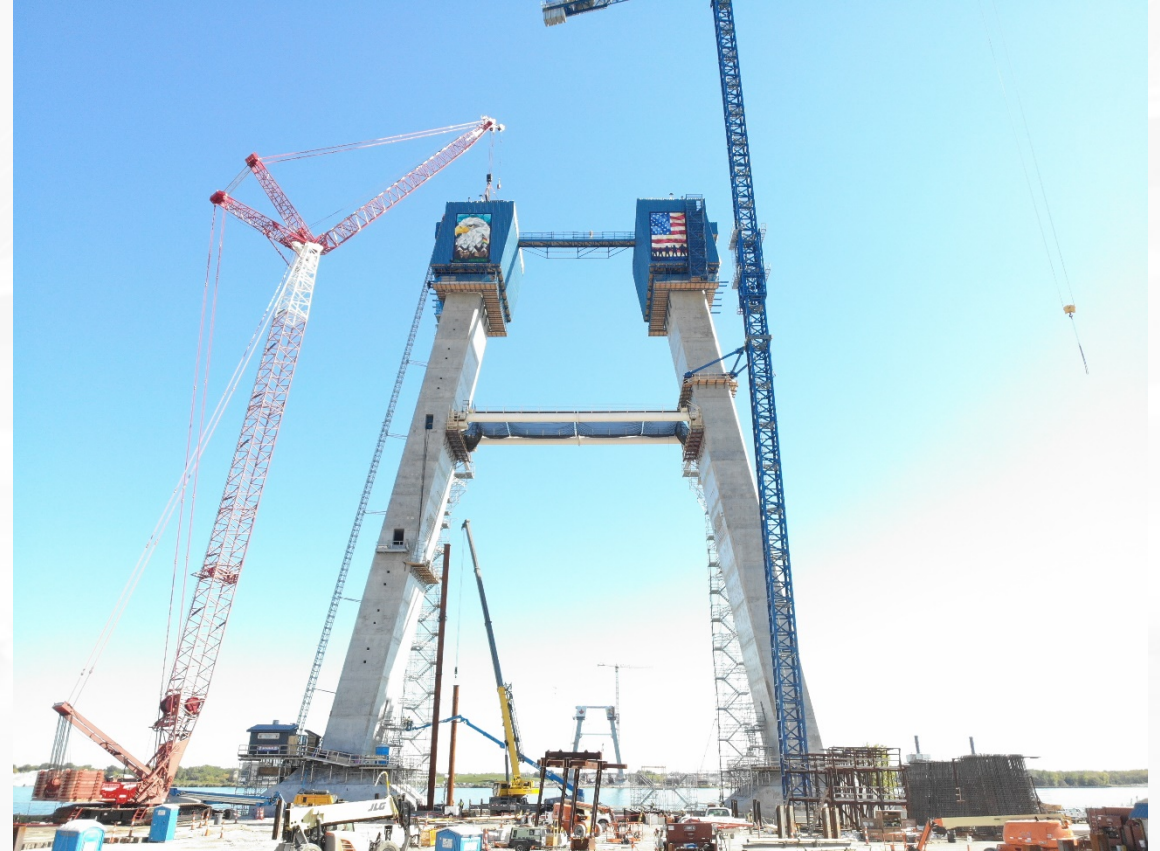
US bridge site tower work
