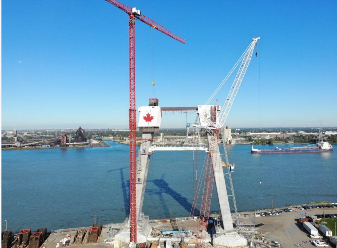
Canadian bridge site tower work
